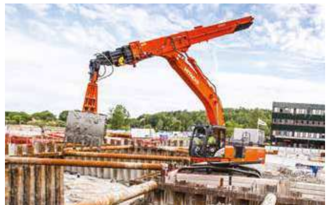
Special application excavators
